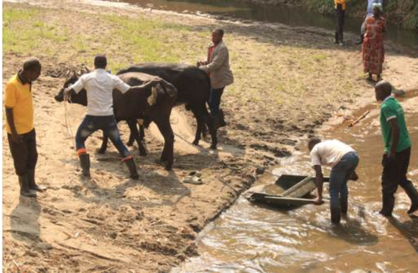
Ox-promoters and operators being trained on how to use oxen for desilting.
